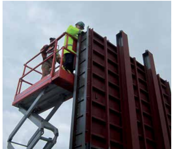
Industry expert inspecting grouting mock-up
